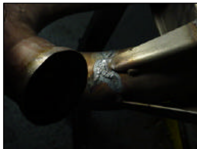
Joe's Cracks Repaired <g>
